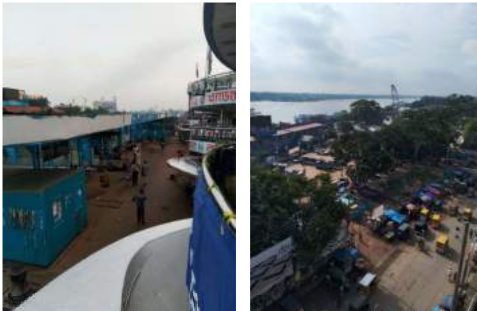
Figure 141. Passenger IWT site at Barishal
