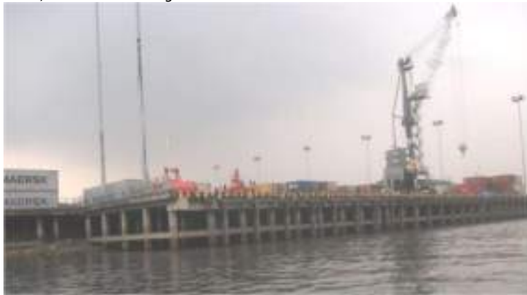
Figure 54. Existing ICT Jetty - Water Side View
