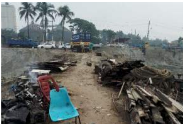
Figure 181. Shasanghat terminal site.
