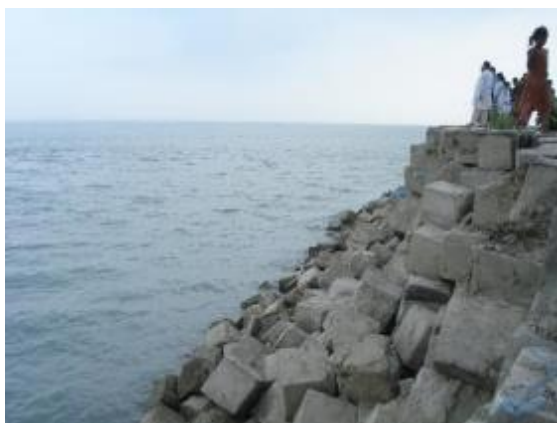
Assorted CC block placed on the bank-slope and low
