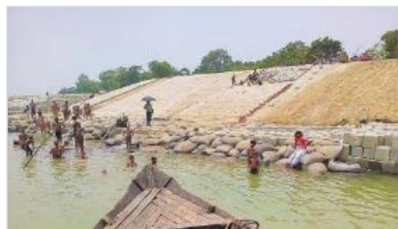
Revetment at Alatuli in Chapainawabganj Sadar upazila
