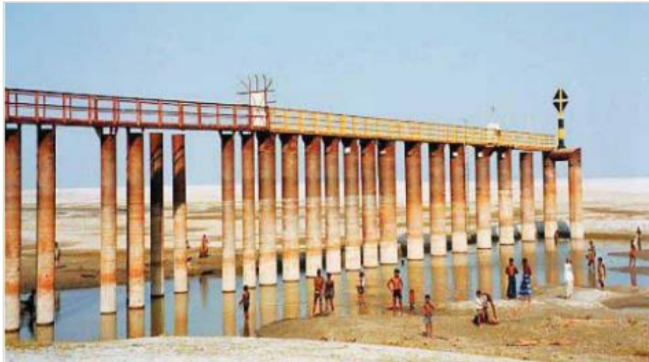
Figure 4.6: Permeable Groyne at Kamarjani of Jamuna River
