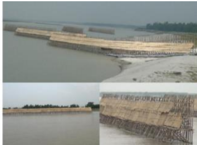
Figure 3.17: Sketch of Permanent-Type Top Blocked Permeable Groyne
